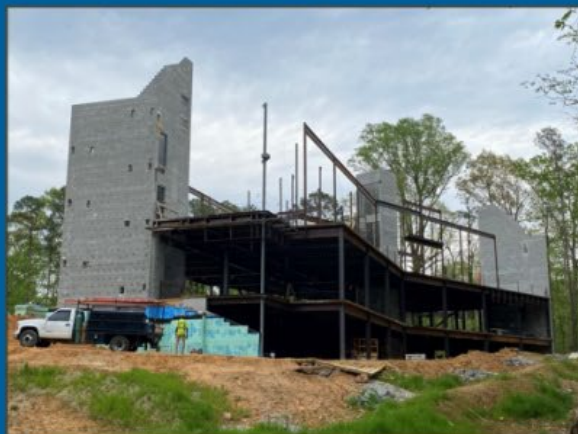
Bldg 3 – Structural Steel Progress
