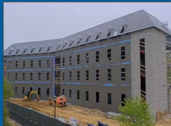
Bldg 2 – Roof Deck / Dormers / Moisture Barrier
