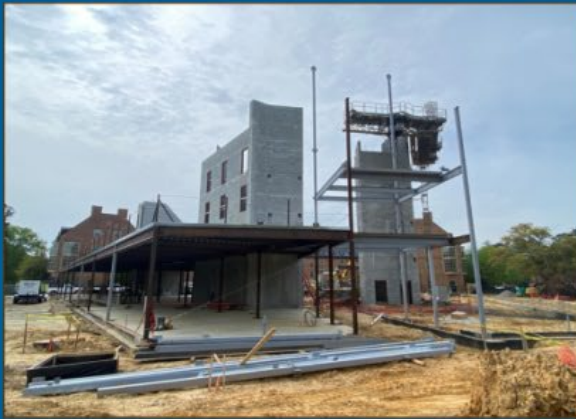
Structural Steel at Entry Portico
