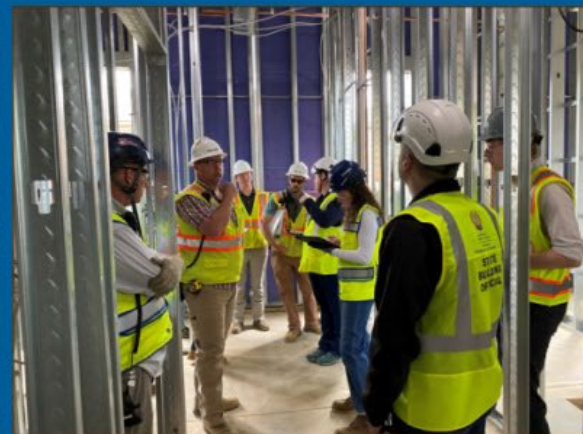
Bldg 2 – DEB Inspection of Level 1 MEP Rough-in
