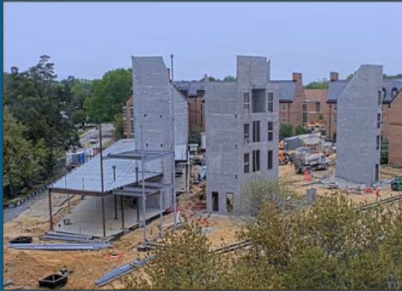
Overall Site – Above Grade Masonry Complete
