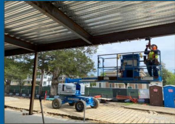
Prep For Metal Framing
