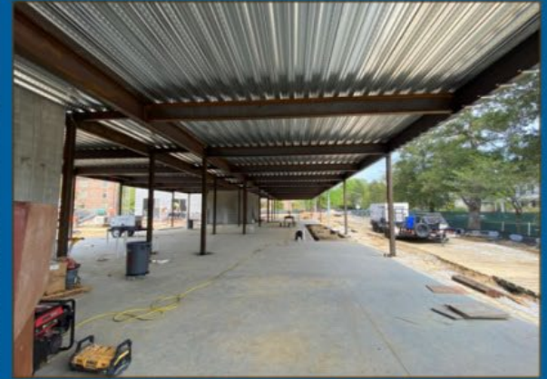
North Wing / Level 1 – Level 2 Deck Overhead
